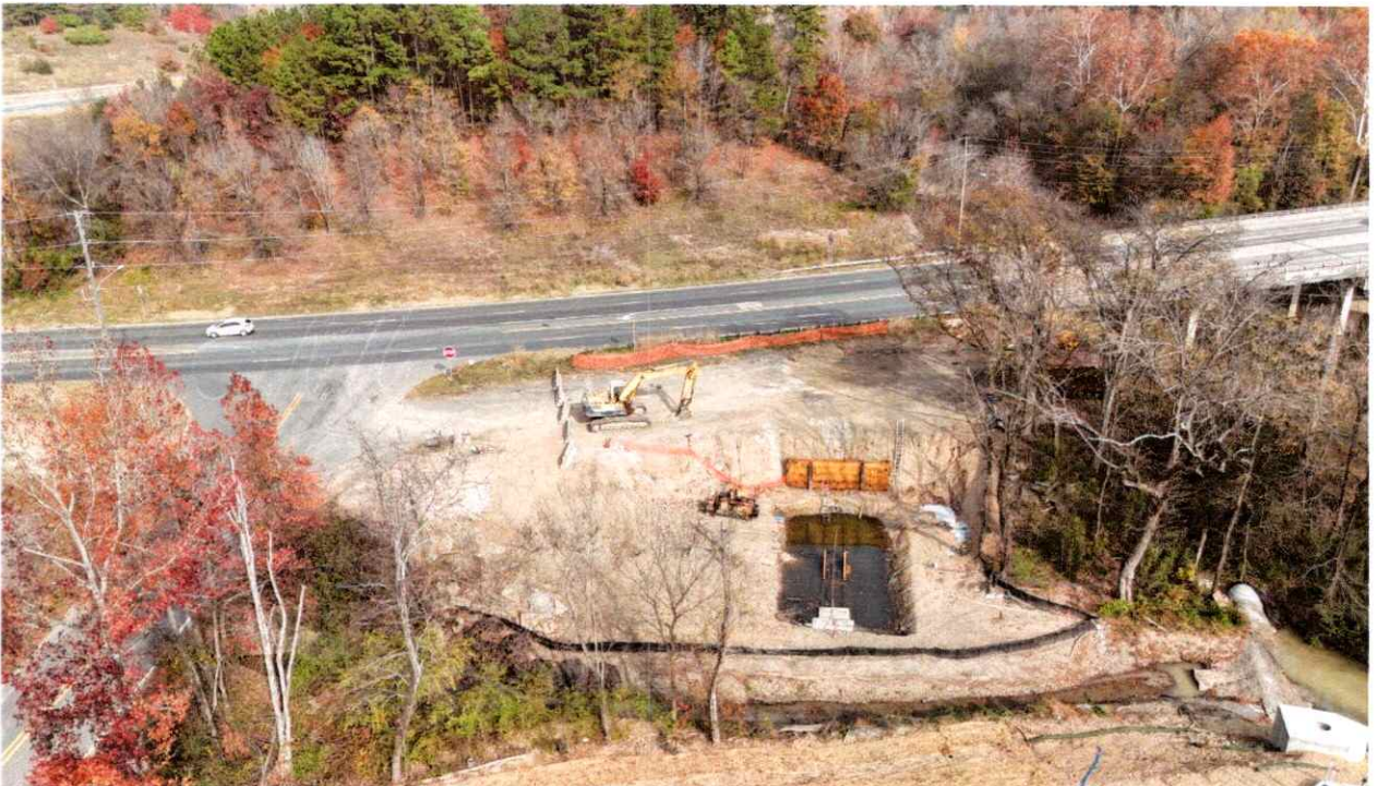
Lower Gulpha Interceptor - Schedule 1 – Bore Site on Highway 270
