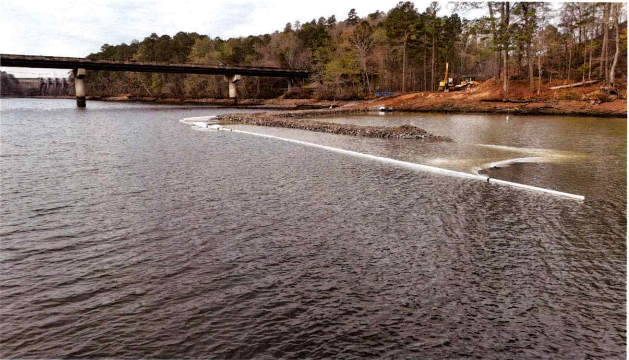
Davidson Drive WWTP Outfall Construction
