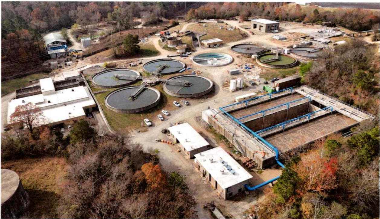
Davidson Drive WWTP Clarifier under construction
