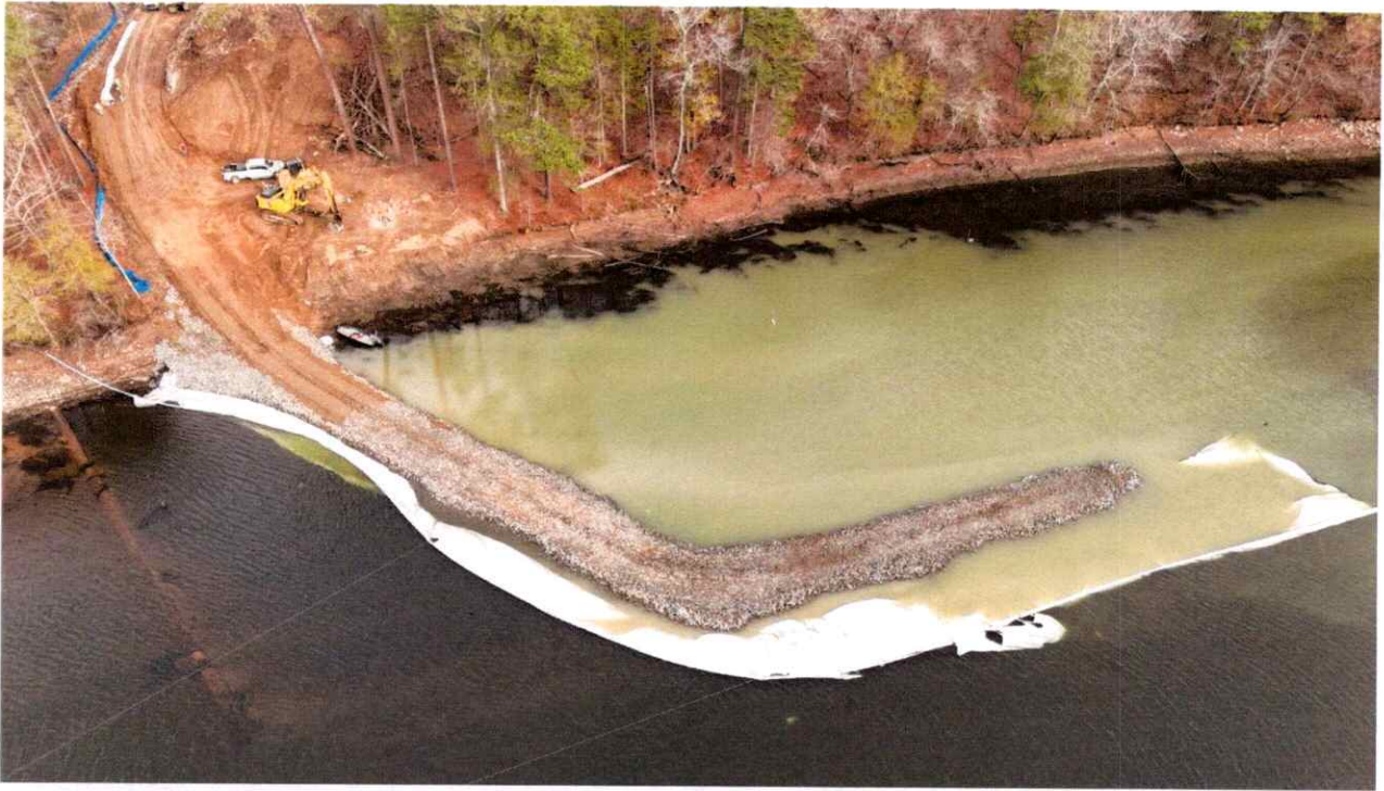
Davidson Drive WWTP Outfall Construction
