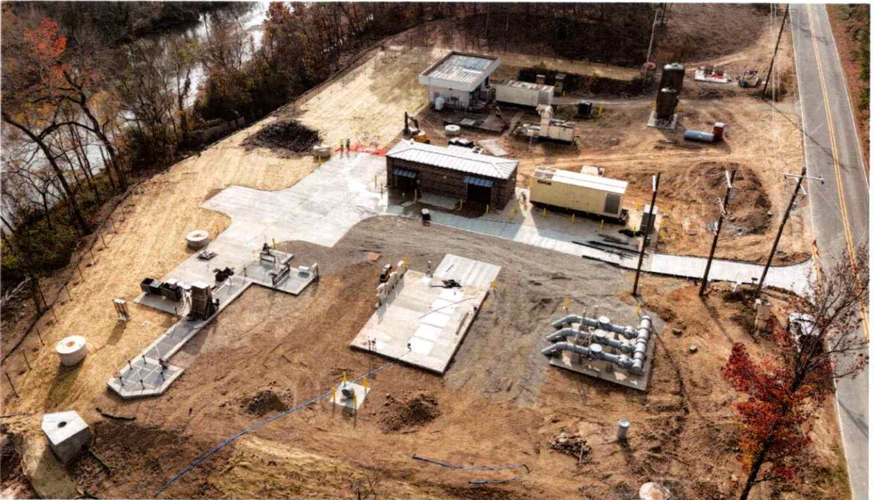
Gulpha Pump Station Construction
