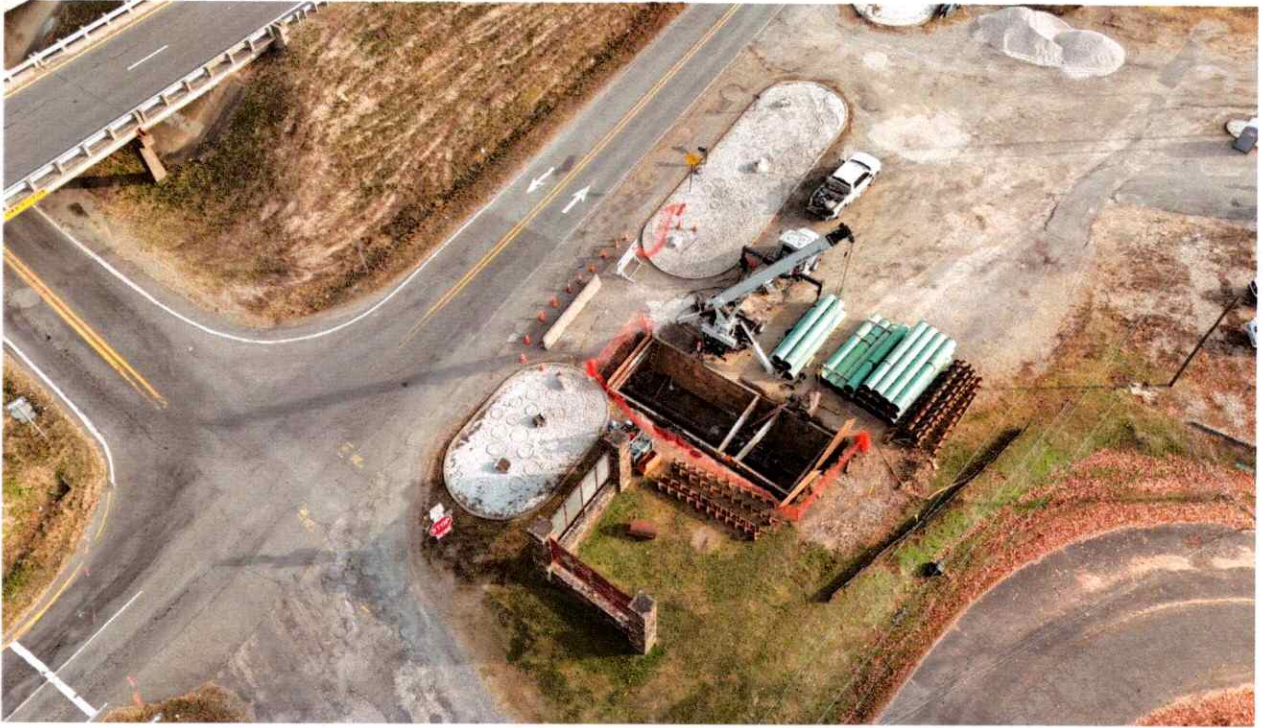
Upper Gulpha Interceptor – Schedule 2 – Bore Site on Highway 70
