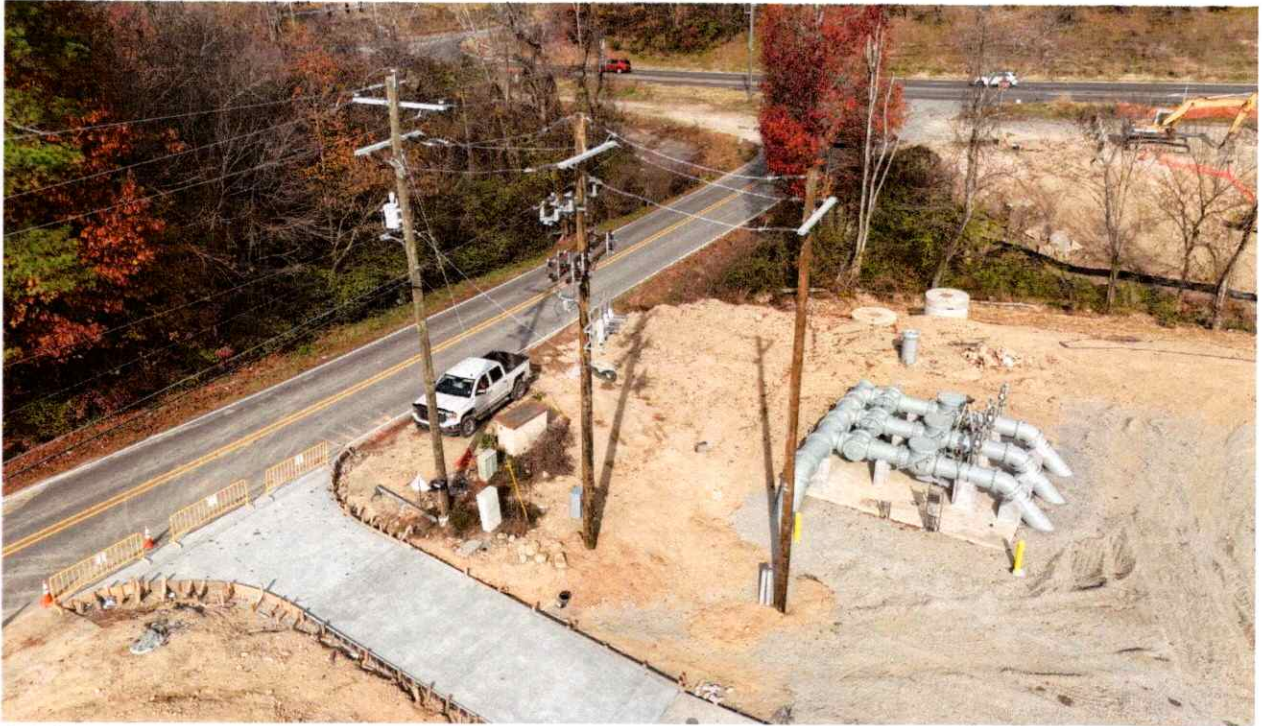
Gulpha Pump Station Construction
